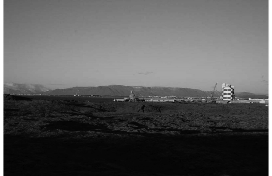
Testing the ground:
