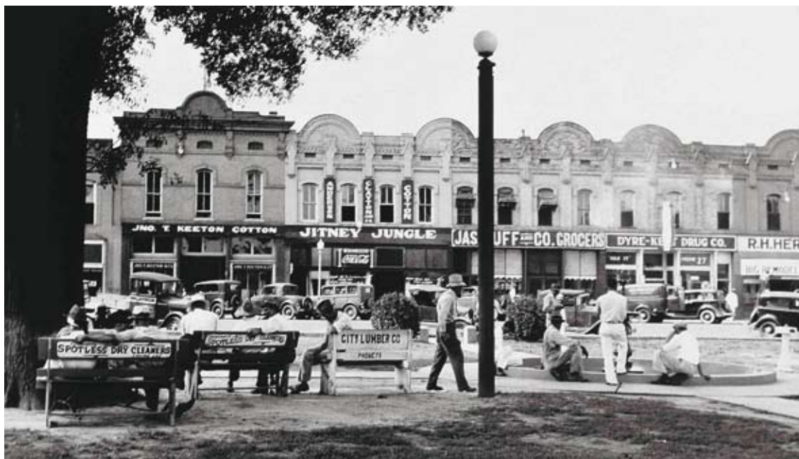
Courthouse Town, Grenada , prior to 1935
