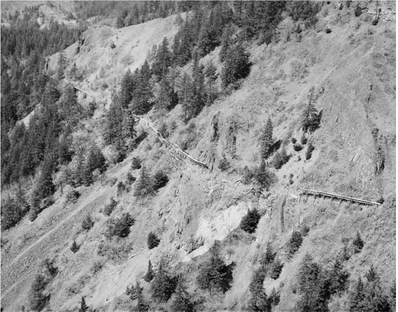
Oblique Aerial View of Collapsed Sections of the Broughton Flume, Skamania County, Washington, 2007
