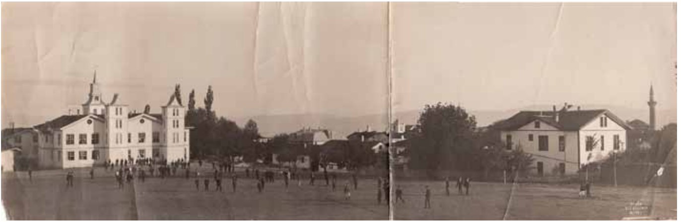
Anatolia College, with Main Building on the left and playing fields in front. Circa 1903.
